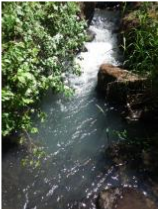
Unit 14.3 – Upstream view of side-channel cascade
